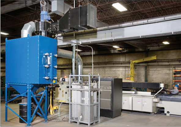
Top mounted PBI Packaged fan installed on a dust collector being used to recirculate the clean exhaust in a manufacturing facility.
