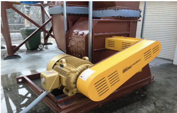
BI Industrial fan serving a baghouse dust collector for a guitar manufacturer.
