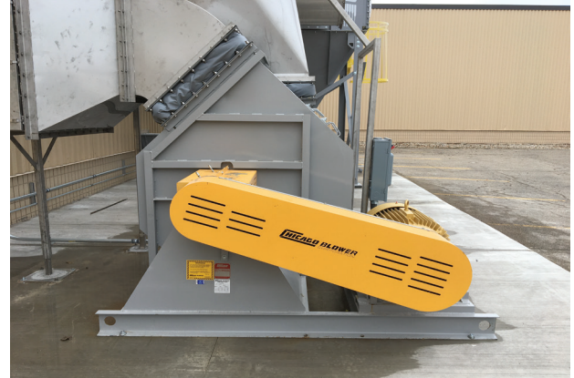
A BI Industrial fan being used as the main dust collection fan on an 18,000 cfm industrial dust collector.
