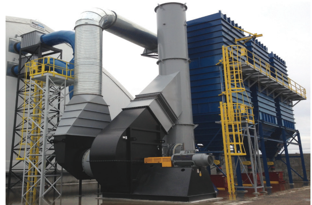
High Pressure Backward Curved fan installed on a dust collector system in Canada.
