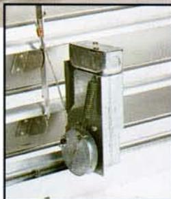
Gravity operated shutters are opened by the fan air stream upon start-up of the fan and
