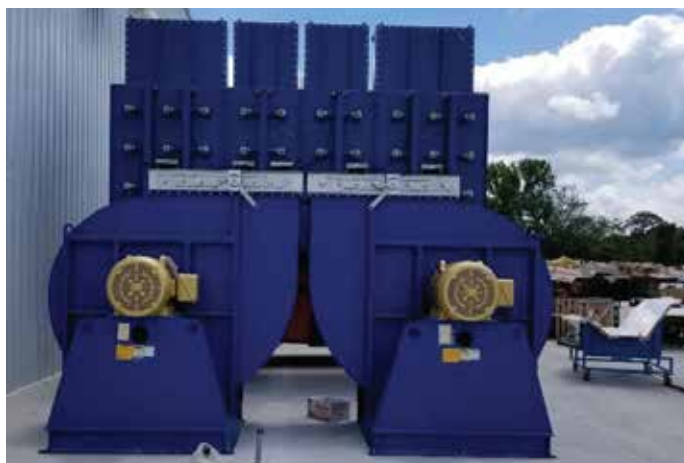
Two PFD fans in a cartridge style collector application used by a boat manufacturer.
