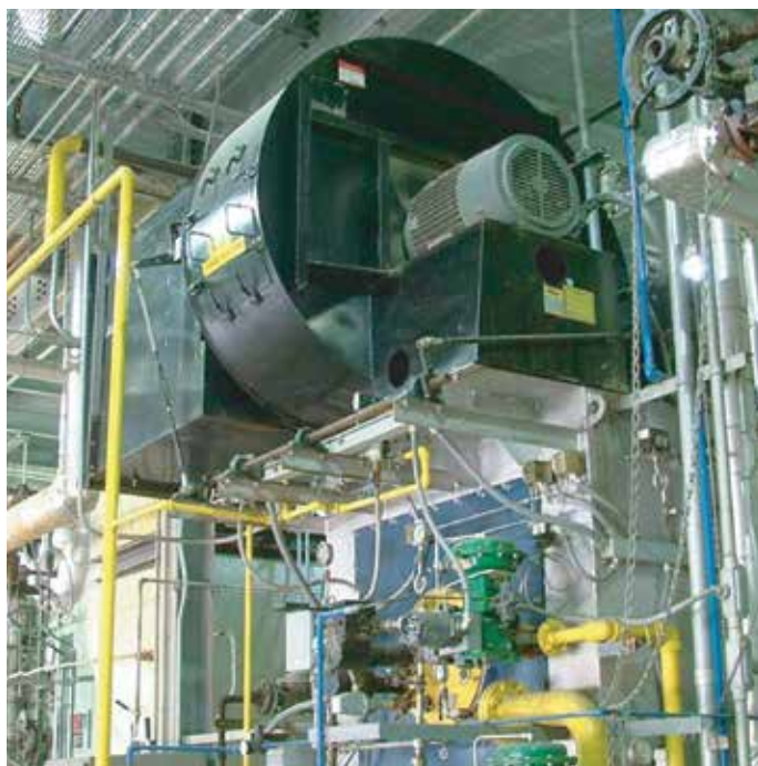
This Packaged Boiler application features a Size 4014 Down-Blast Arrangement 4 fan mounted to a wind-box.
