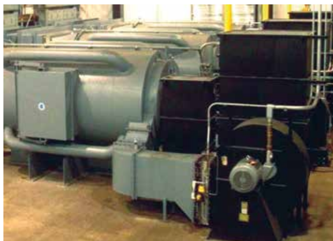
Burner installation utilizing three Size 2700 A/4 PFD fans.
